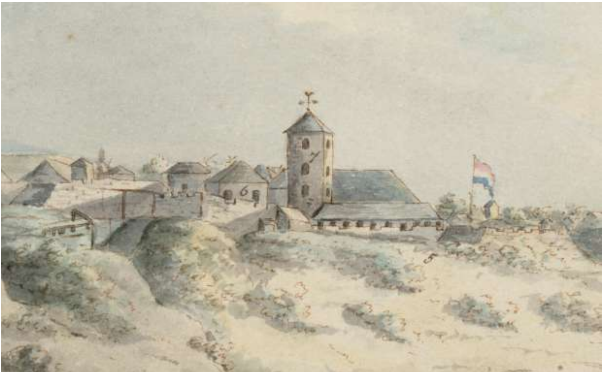
Figure 4 Detail of Upper Town Oranjestad from A. Nelson Watercolor (1774). The number five depicts Fort Oranje and the number six depicts the government offices inside the fort.
